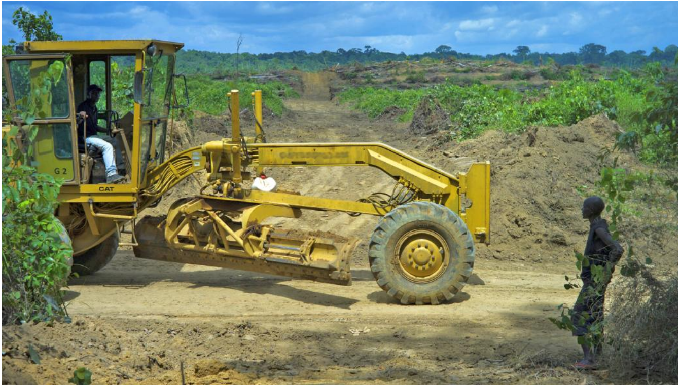
Land being cleared and replanted with oil palms at the Butaw plantation in Sinoe County, Liberia (2014). Anna Fawcus/Oxfam America
